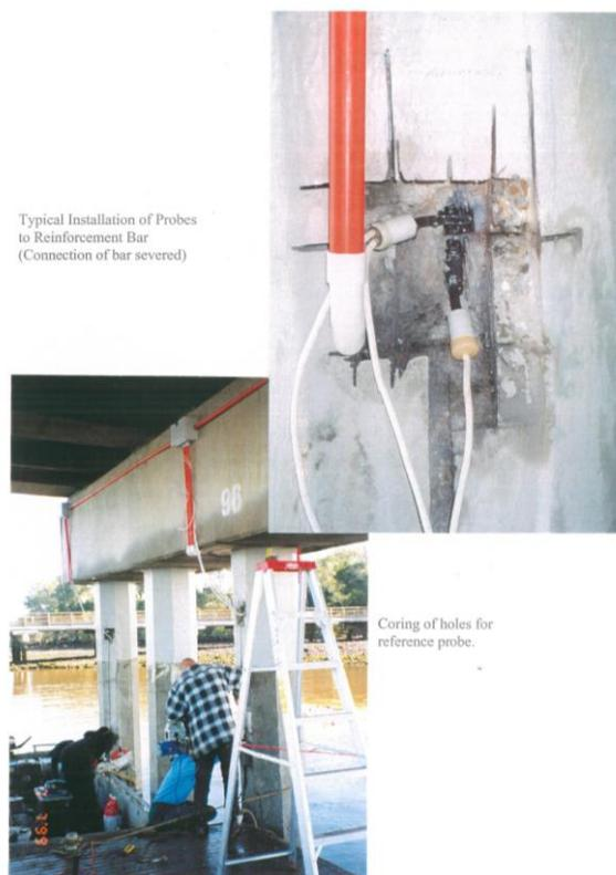
Figure IV View of LPR probe locations
