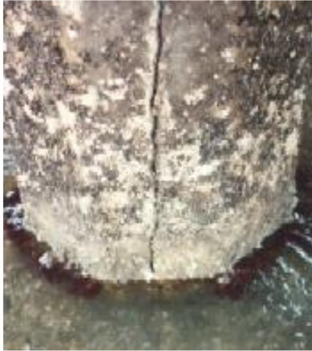
Figure II View of vertical crack in prestressed piles
