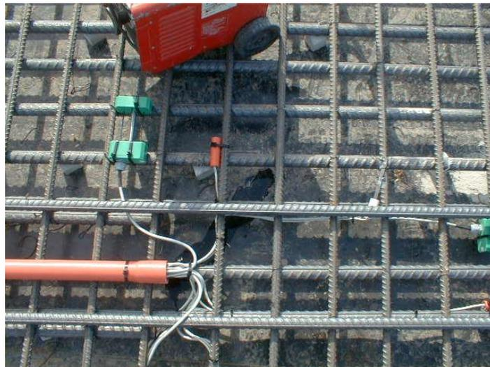
Figure X View of LPR probe installation
