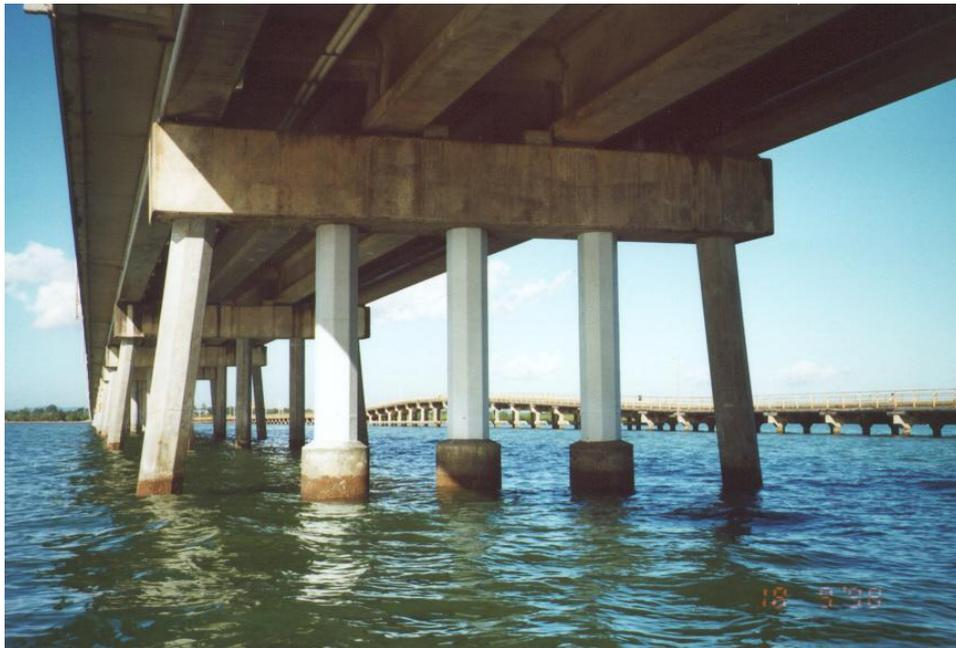
Figure III View of Concrete and Fibre Composite Encasement of Piles
