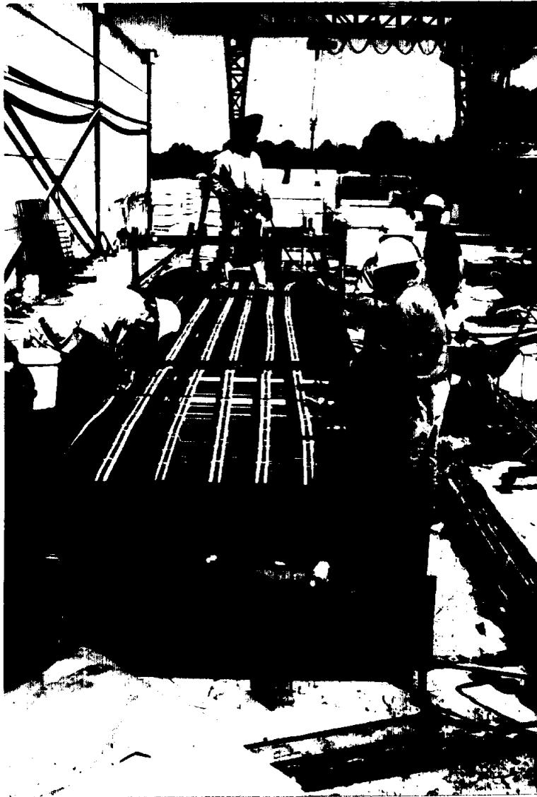
Photo n° 4: walkway anode installation.
