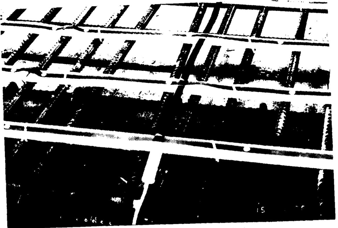
Photo n° 3: detail of walkway anode installation.
