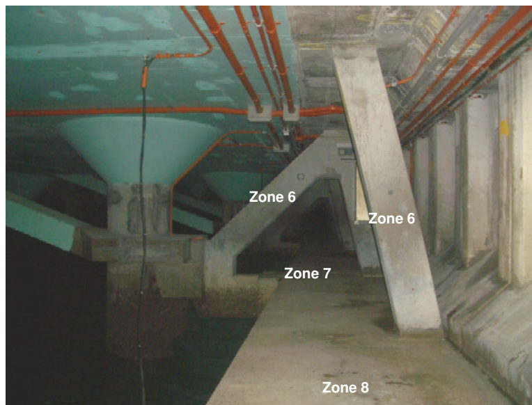
Figure 2: Electrical Zoning of System
